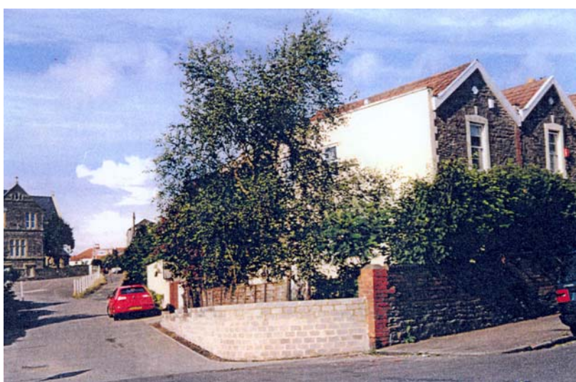
Mrs Blackwell supplied photograph showing new wall surrounding verge, summer 2000
