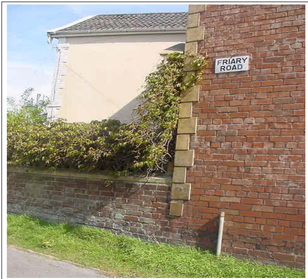
SITE VISIT 1.05.2003 – Friary Road nameplate on side of No. 122 Egerton Road.
