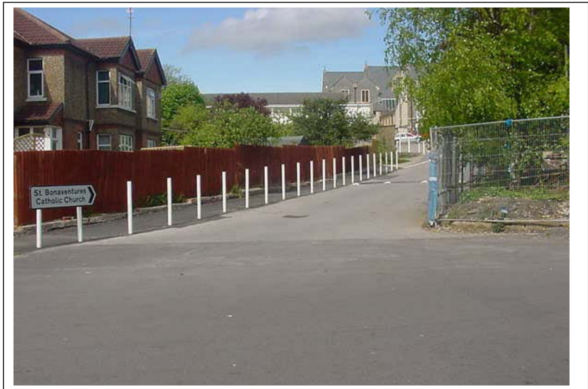
SITE VISIT 1.05.2003 – ‘New’ footway and Heras fencing at the Berkeley Road end of Friary Road.
